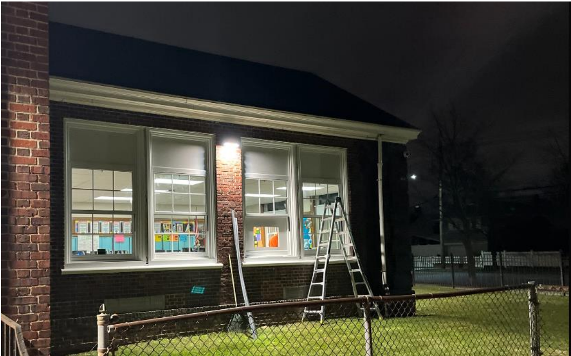
Hempstead UFSD – Phase 1 Window Replacements – Jackson Main ES
