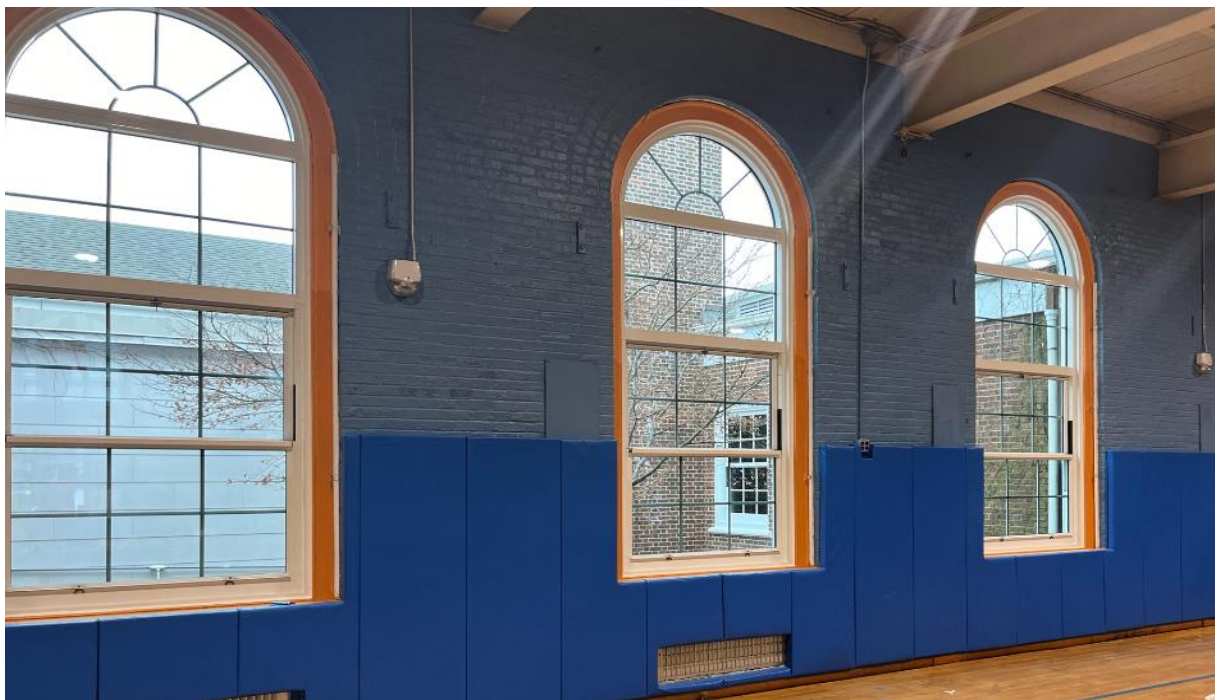
Hempstead UFSD – Phase 1 Window Replacements - Jackson Main ES
